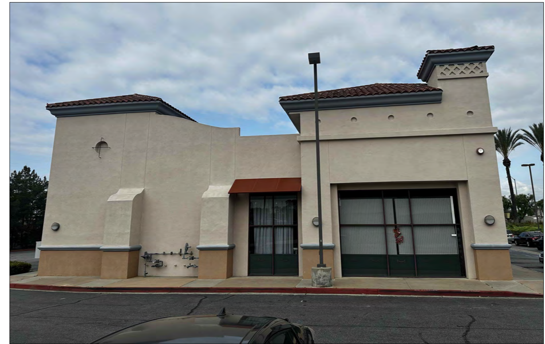
(EAST) BUILDING SIDE 1
