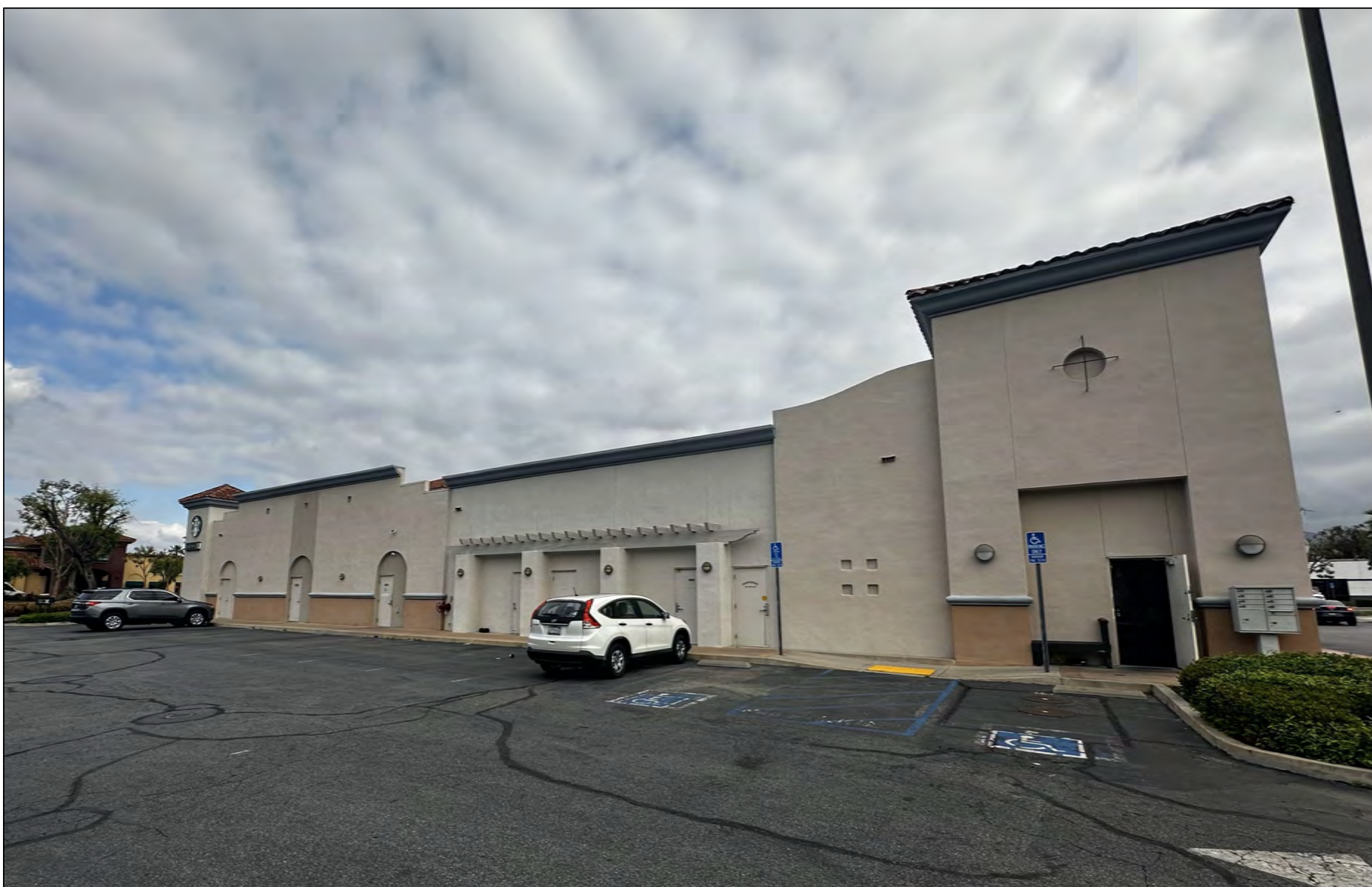
(SOUTH) BUILDING REAR 5
