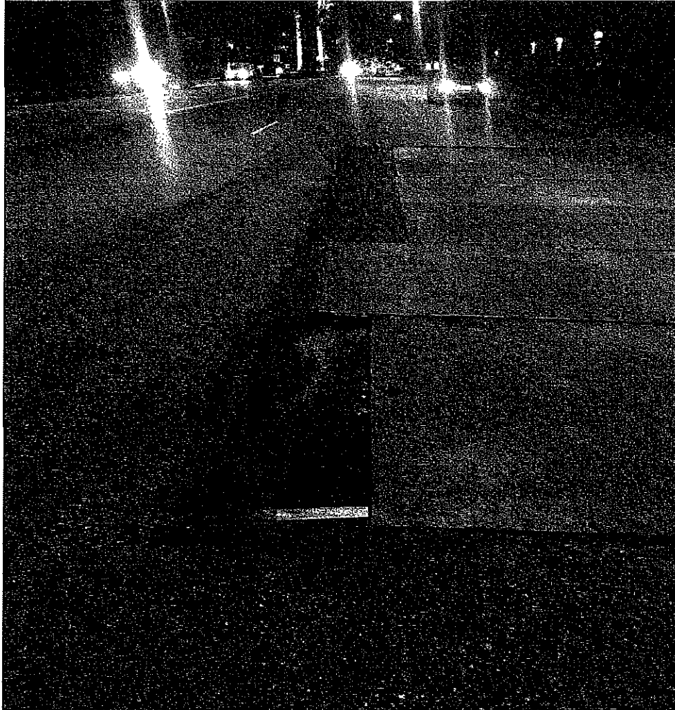
Hazardous steel plates on Arrow highway
