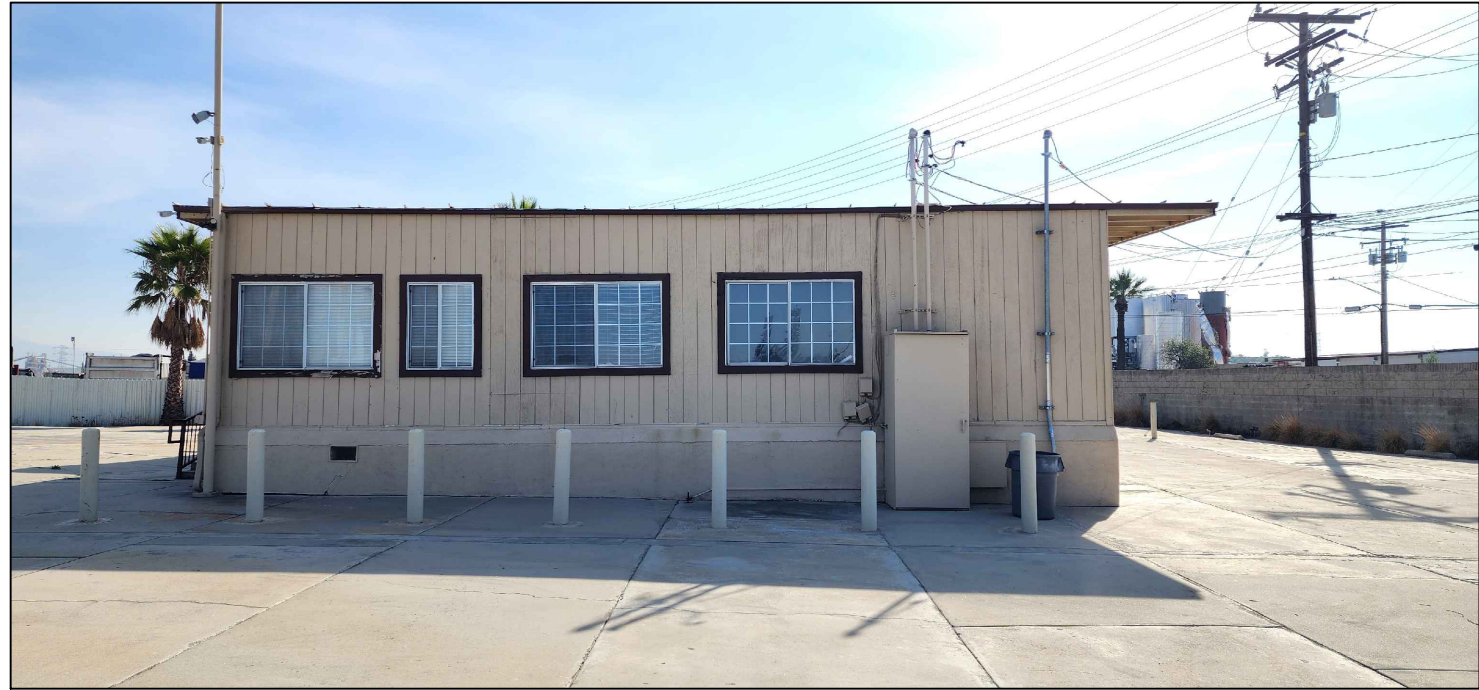
WEST ELEVATION - EXISTING BUILDING #2 TO BE REMOVED
